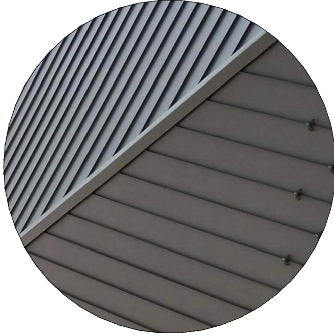
4. STANDING SEAM ROOFING
