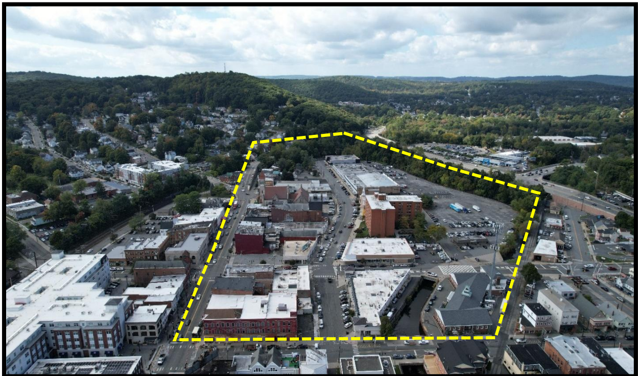
Figure 3 ~ Aerial drone photograph of Bassett Highway district, looking west (taken by John McDonough Associates 10/3/ 2024)
