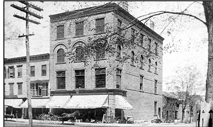
Figure 1: Historical Photo of the Former Berry Hardware Store
