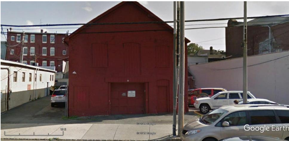
Figure 24: Building on Lot 8 is a two-story brick storage building with boarded windows and is owned in common with the mixed-use building on Lot 7. Google street view is dated August of 2018.
