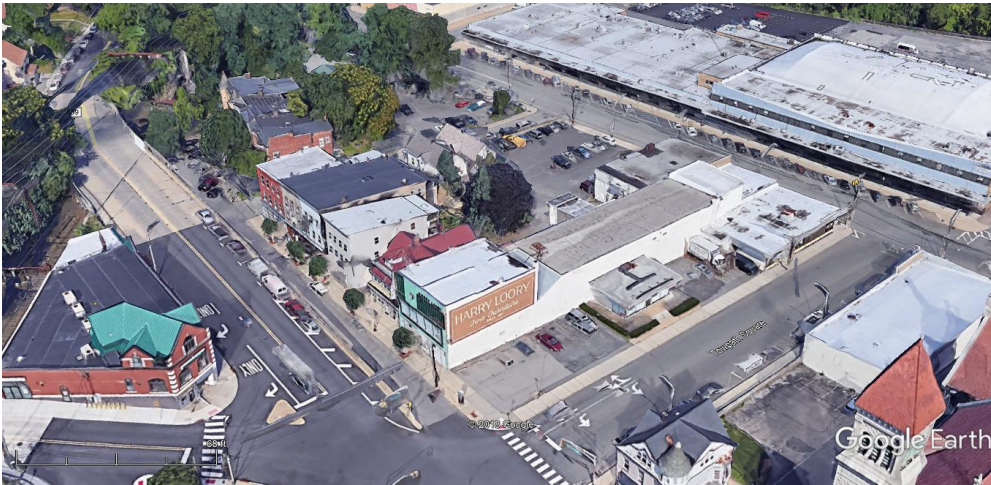
Figure 16: Birds eye Google Earth view of Block 1205, with the most significant building, the Harry Loory Furniture Store visible at the corner of East Blackwell Street and Towpath Square (Prospect St.). Image dated August 2018.
