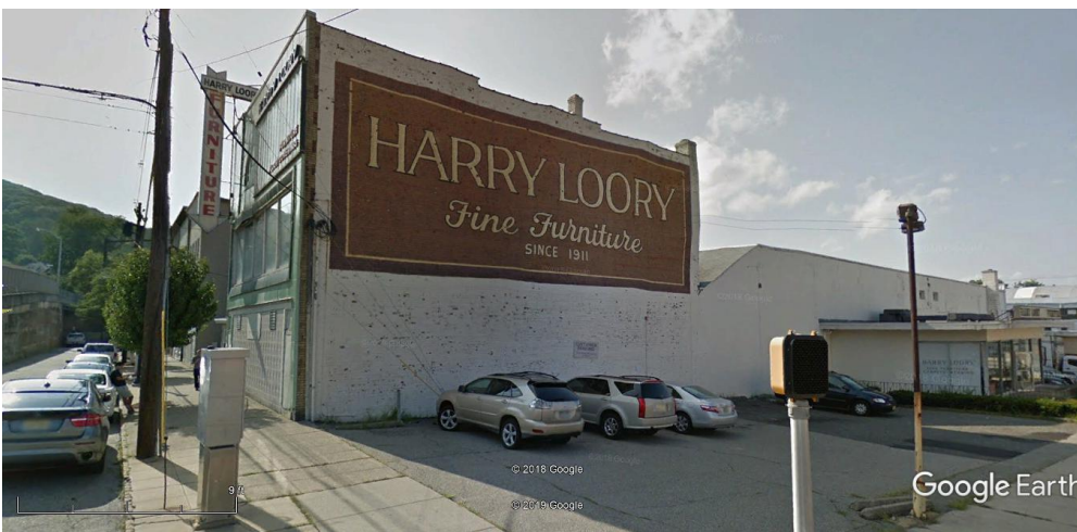
Figure 17: A Google street view of the Harry Loory Furniture Building on Lot 2, with the parking in the foreground on Lot 1, dated August of 2018.
