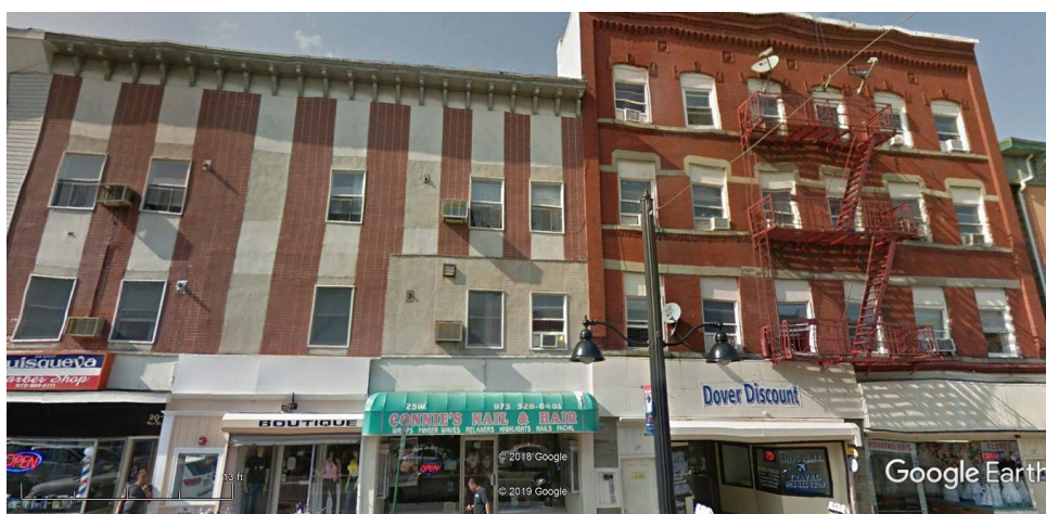
Figure 23: Buildings on Lot 6 (right) and 7(left). The 4-story building on Lot 6 has retained its historic façade, in contrast to the 3-story building on Lot 7.
