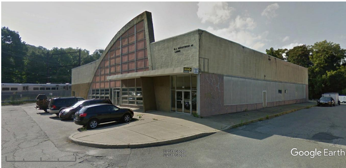
Figure 11: Building on Block 1201, Lot 6.01.
