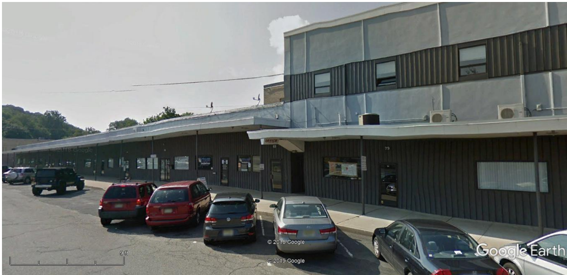
Figure 9: Google Earth streetview of building on Lot 6 taken in August of 2018.
