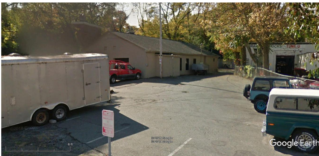
Figure 15: Google street view of building on Lot 2 (4-6 Dewey Street) dated August 2018.
