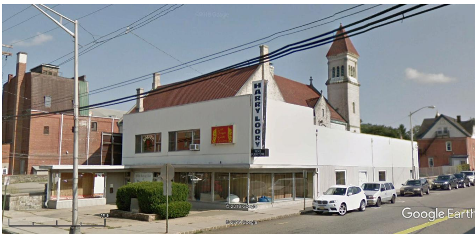
Figure 26: Google Earth street view of the building on Block 1206, Lot 16, occupied by Harry Loory Fine Furniture on the ground floor and a karate studio on the second floor, dated August of 2018.
